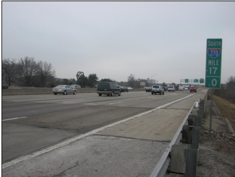
Southbound I-270 Marine Avenue bridge
